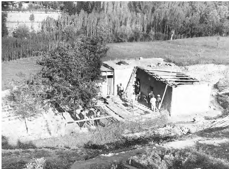
Fig. 5. The dighouse being built at the foot of the mound.
